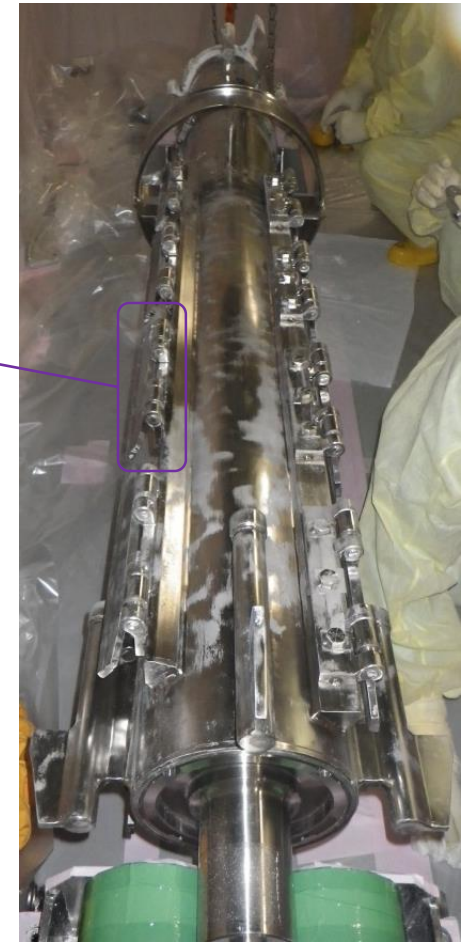
CSS dryer shaft after UEC
