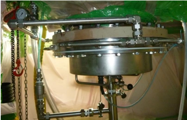
Field installation of lower UEC transducer assembly
